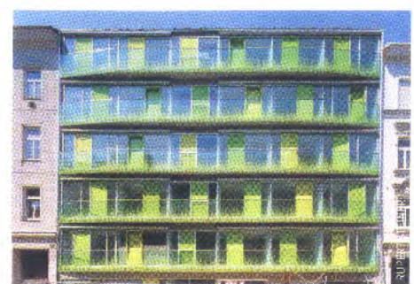
↑ BLOCK OF FLATS, LEEBGASSE, VIENNA (2004) Filling the vacant lot with artificial nature sets the building off from its neighbours. All rooms have access to balconies and feature deep windowsills that can double as seating indoors.
