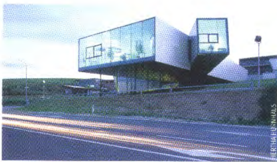
↑ VIT SHOWROOM, ASPERHOFEN (2003) Instead of terracing the sloping lot in the business park, the industrial building was stood on thin stilts. One "trunk" serves as the entrance to the showroom for prefabricated conservatories, the other contains the office. (See also A10 #1)
